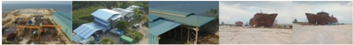
LINTECH SEASIDE FACILITY ( LSF )
